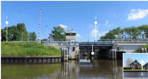
Figure 2. Overview of several measurement positions necessary to determine the bridge correction conform the measurement protocol from the National Public Works and Water Management Office (1= reference point beside the road; 2= point above the bridge; 3 = point below the bridge; 4= immission point in the direct environment)
